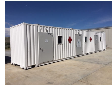
SELF CONTAINED ISOLATION UNIT (SCIU) SUBLETTE COUNTY, WY
