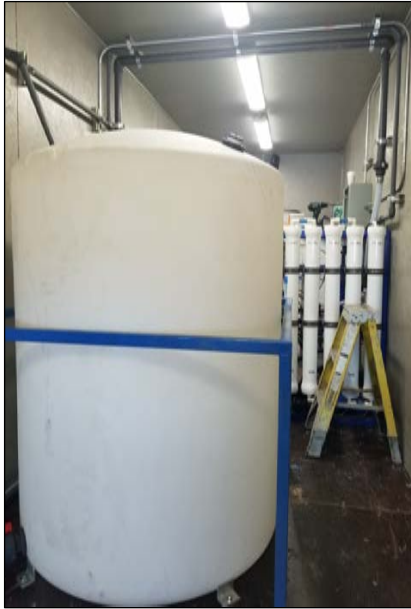
Water Storage, Filtration System and Hot Water Heater housed in CONEX Container.
