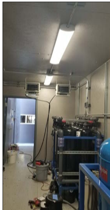
CONEX Box with side openings and divider walls in construction progress including plumbing, electrical, and divided rooms.
