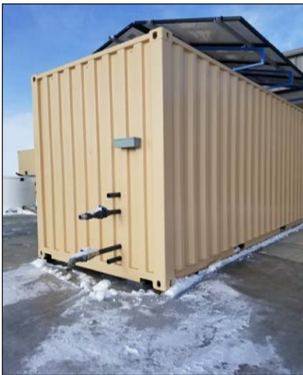
Left: Exterior of ESI Rain Harvest System showing Utility Hub points.
